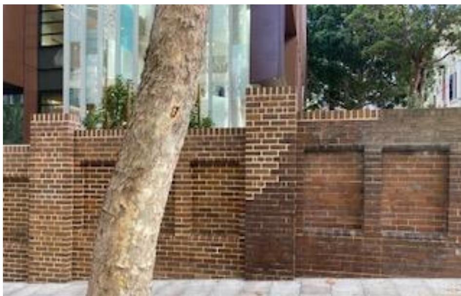
Figure 6.1 A section of the c1920s brick wall outside Monte Saint Angelo Convent at 128 Miller Street, North Sydney was disassembled for three months in 2023 during adjacent building works, and then reconstructed with a fine result.
